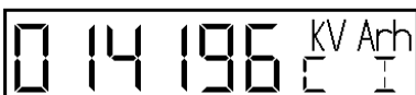
Cumulative total register for kvarh lag, in this case showing 14196 kvarh. (Only on model EN305).
